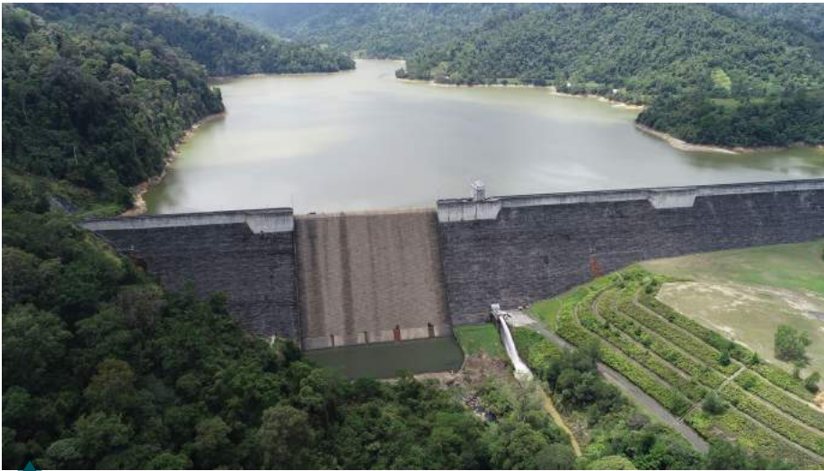
Sultan Azlan Shah Dam, Perak, which is the first Roller-Compacted Concrete (RCC) Dam in Malaysia, engineered by Angkasa-GHD Engineers Sdn. Bhd., now known as Angkasa Consulting Services Sdn. Bhd.
