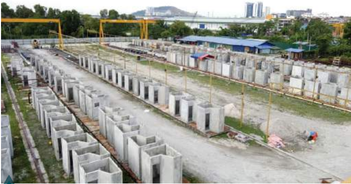
PBUs being assembled at Setia Precast's USJ Yard
